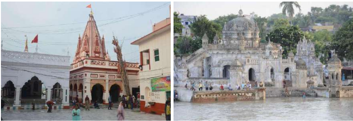
Figure 19 a) Burhanath Temple with a central Garba Griha topped by a Shikhara and a pradakshina path circumscribing it b) Radha Krishna Temple at Siddhi Ghat, Bhagalpur with borrowed elements from Islamic architectural styles. Source: https://bestplacesofindia.com/bhagalpur/ Accessed online on 21.01.2021
